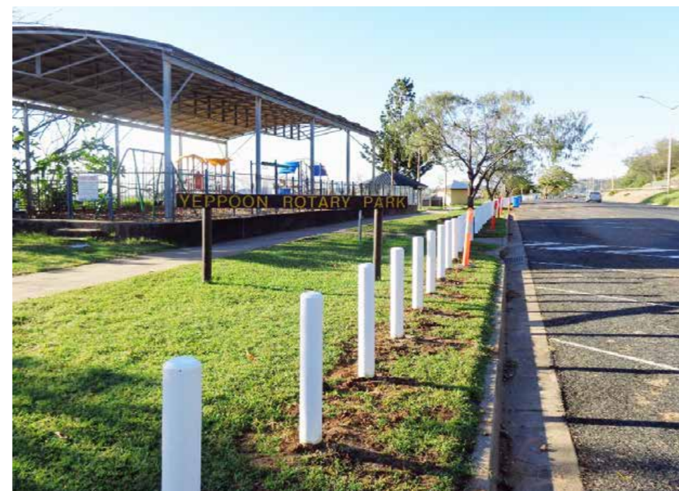
Photos clockwise from top: A prisoner constructing foreshore safety barrier fencing | Low security prisoners cleaning up one of the nominated public parks | Bollards installed by prisoners along the boundary of Yeppoon Rotary Park | Field Supervisor, Peter Cronin assisting in the clean up.
