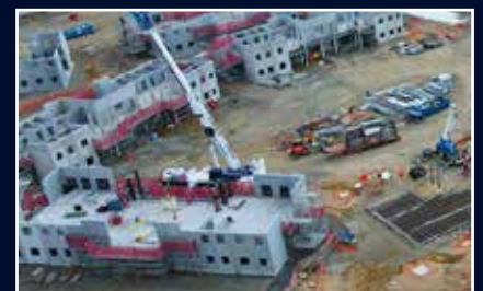
New milestones for new Southern Queensland Correctional Precinct Stage 2 Page 13
